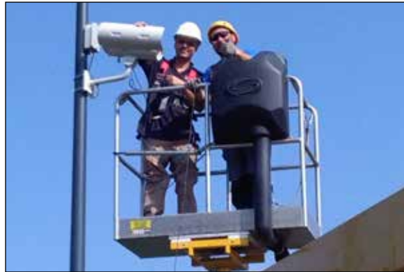
Technicians installing security cameras.
